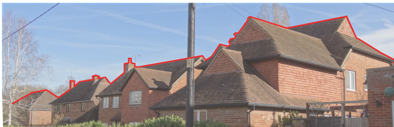
Figure 26: A varied, interesting roofline with a consistent ridgelines and material use and chimneys which add a focal point element for views.
