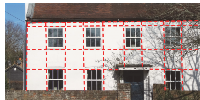
Figure 25: Example of a well-proportioned facade in Eversley that evenly aligns fenestration and utilises smaller upper windows.
