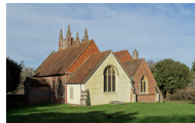
Figure 08: Grade I listed Church of St Mary of medieval origin, located within the Church Farm Conservation Area.
