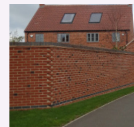
Overly high walls
