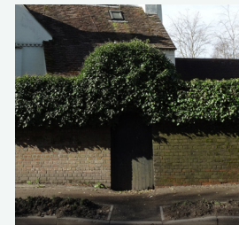
Mixed material wall
