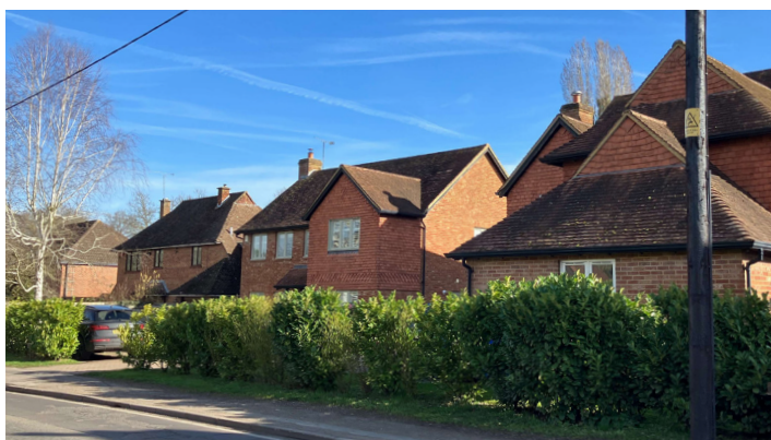
Figure 21: A row of dwellings featuring a uniformity in traditional materials but an interesting variety in roofscape and built form.
