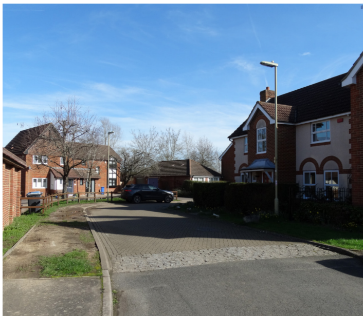
Figure 14: Grensell close utilises a variety of architectural detailing and building orientations to create a more interesting streetscape.
